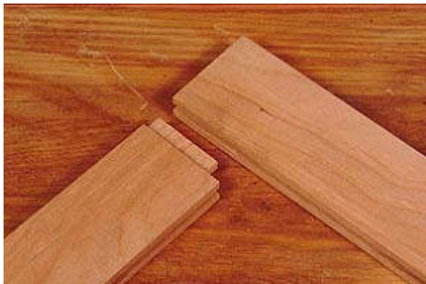
Photo 4- The finished joints will appear as shown. This is a small joint, but then it's a small door. Still, it's important to get a good fit between the tenons and the mortise grooves for a good glue bond.
