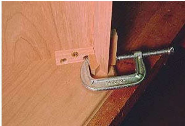
Photo 19- Two little custom fitted door stops, one at the top and one at the bottom, will prevent the door from swinging in too far.
